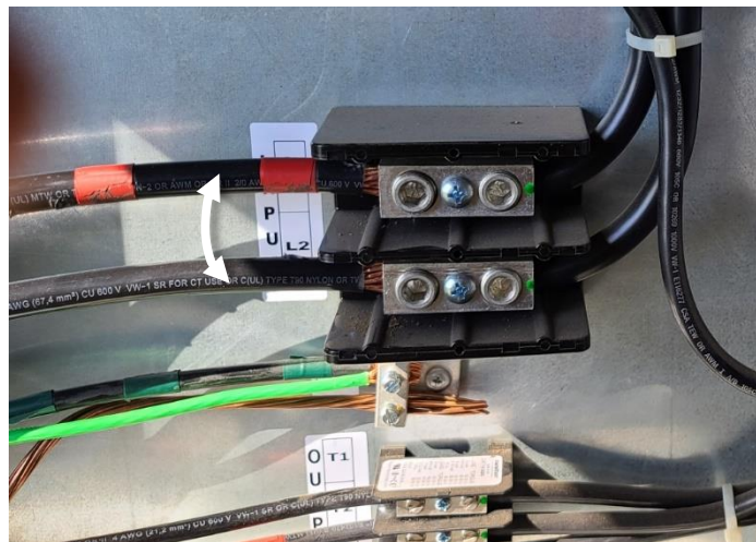
Figure 1 – Rotating input power cables can often resolve LED flicker
