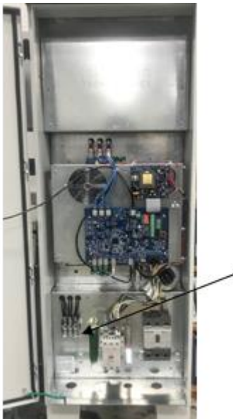
Figure 7 – Signature Series Output Power Terminal Locations
